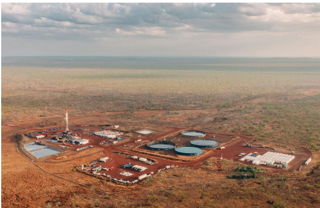
Figure 1: Drilling operations completing in EP 161, November 2021
