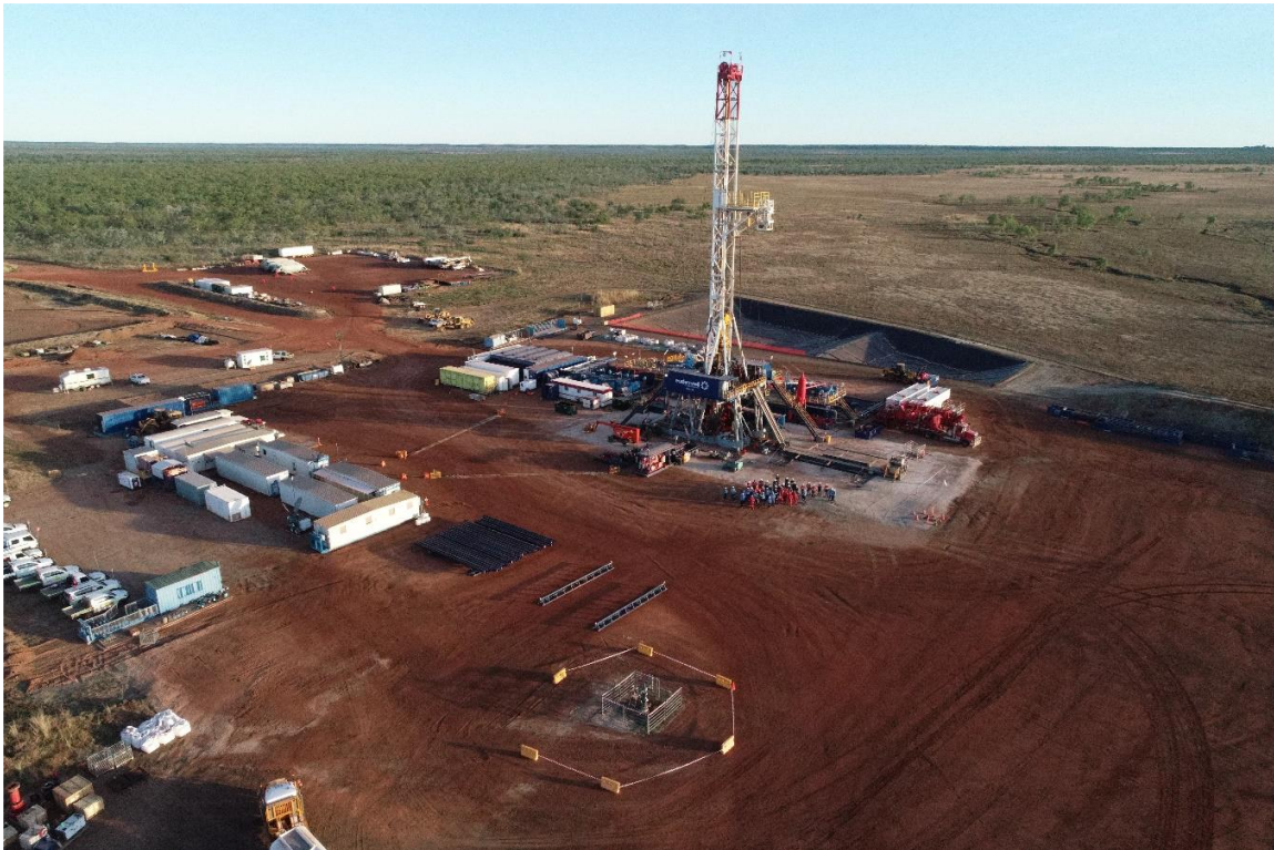
Figure 1: Current drilling operation at EP 161 Tanumbirini 2H
